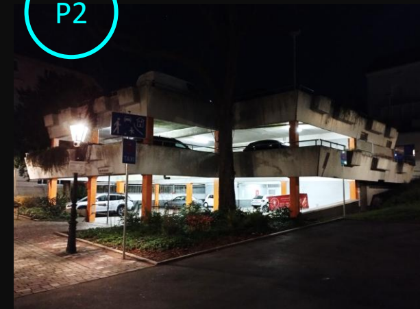
Parkpalette Turmstrasse (Bestandssituation)
